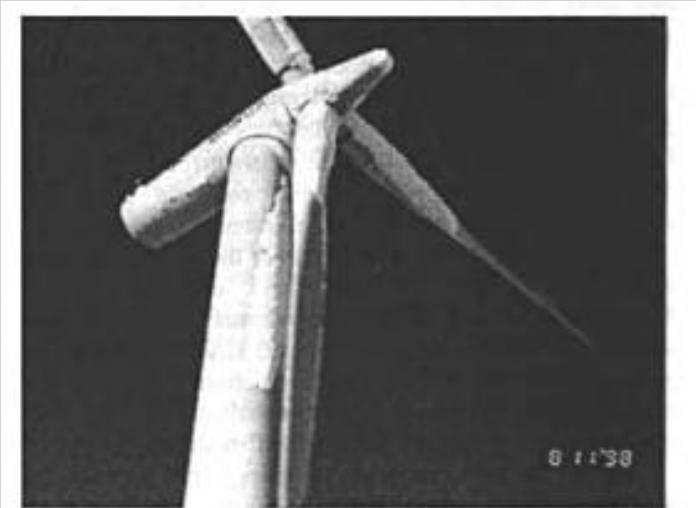
Figure 4. Bonus 600 kW wind turbine provided with the blade heating system on the top of Lammasoaiivi Fell in the most Northern parts of Finland.
